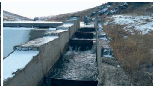
Fig. 2.3. Water intake unit and fish passage of Argichi SHPP
