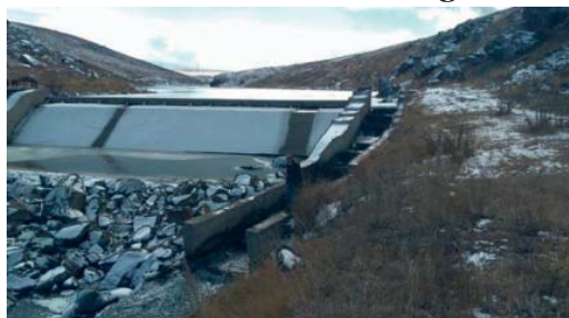
Fig. 2.3. Water intake unit and fish passage of Argichi SHPP
