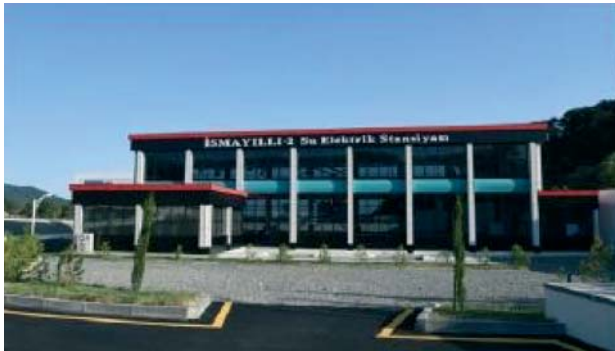
Fig. 2.10. Ismayilli-2 hydroelectric power plant with an installed capacity of 1.6 MW
