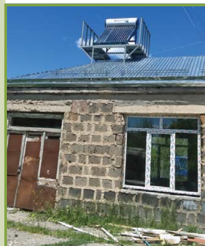
Solar water heater installation on the roof of Vanatur kindergarten
