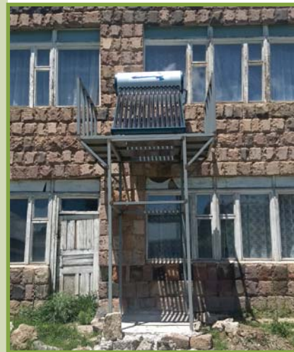
Installation of solar water heater on the roof of Jrarat kindergarten
